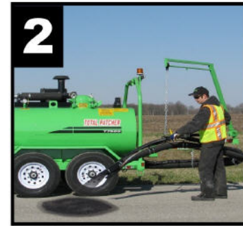
2 Apply tack coat to area to be repaired
