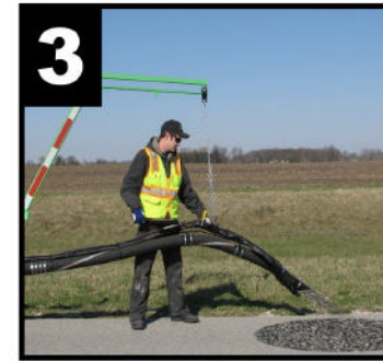
3 Apply aggregate/emulsion mixture - you're done!
